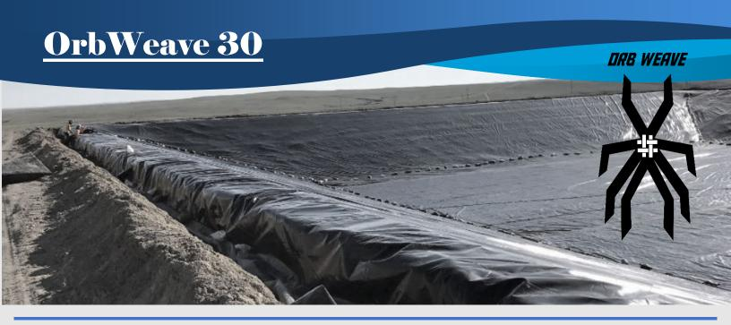
OrbWeave 30 is a multi-layer reinforced 12.4oz/yd² geomembrane ideal for medium and heavy-duty applications. OrbWeave 30 is the industry leader in quality and strength. An extremely chemical and puncture resistant geomembrane with light weight HDPE woven skrim core with OrbWeave JAG technology.
